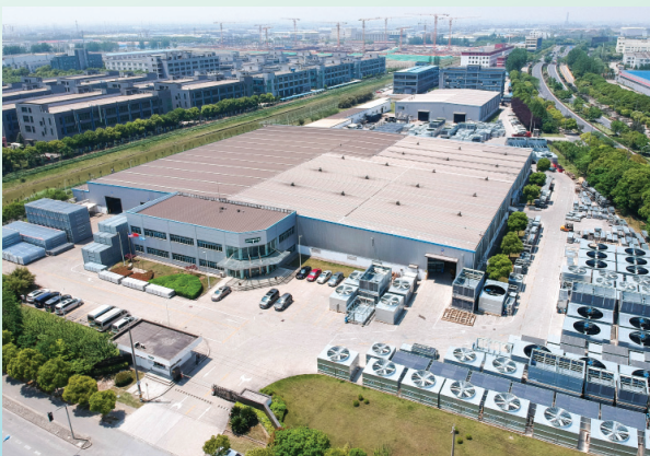
EVAPCO's wholly-owned factory in Shanghai, China
