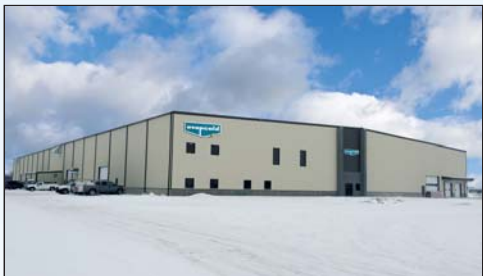
Evapcold Manufacturing, Greenup, Illinois
