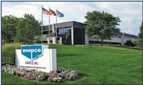
EVAPCO Global Headquarters, Taneytown, Maryland USA
