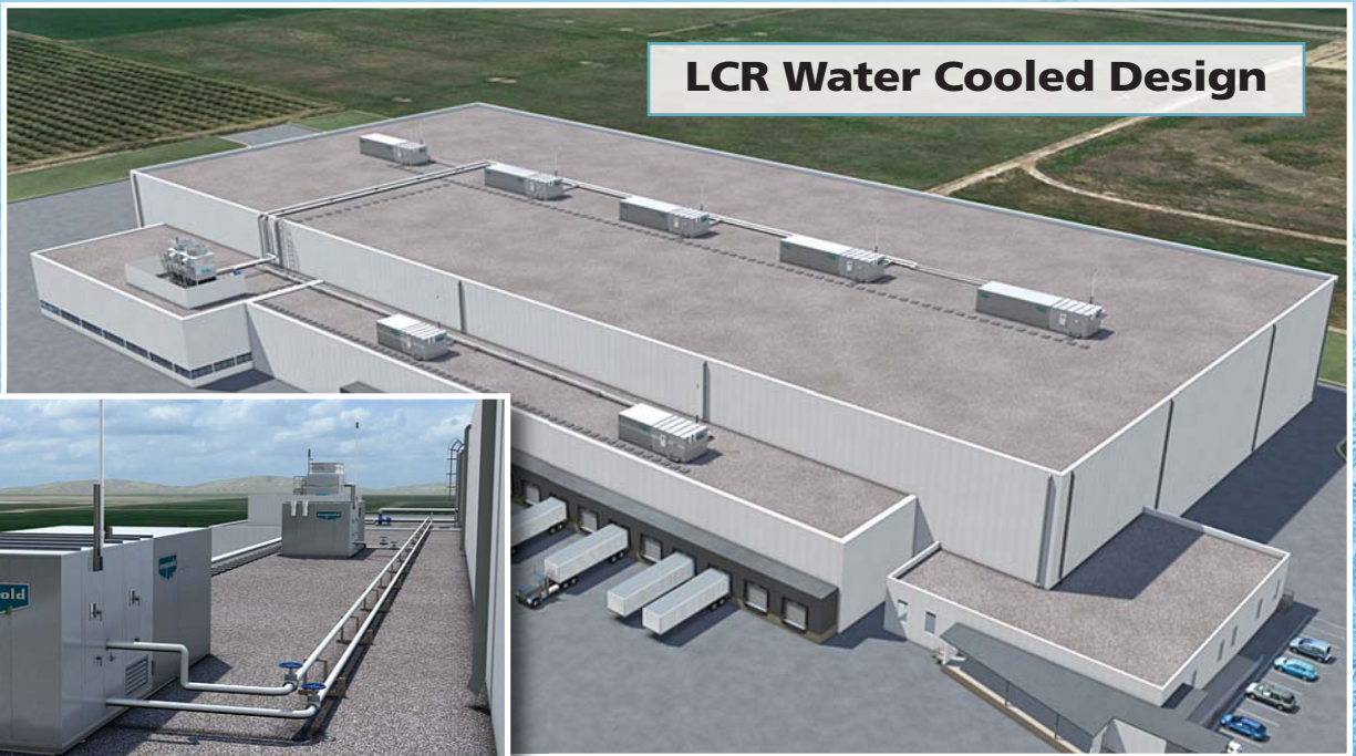
LCR units shown with cooling water piping from cooling tower or fluid cooler
